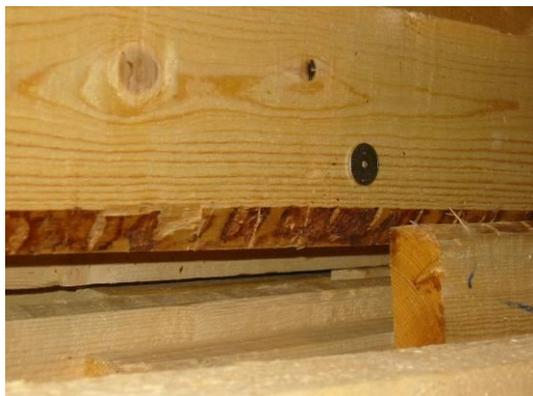
**Image 1**– Wane on edge of board is not regulated.
